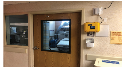
FIGURE 1 Conversion of a typical medical-surgical patient room to a temporary negative pressure patient room. (Left) A typical medical-surgical patient room may be quickly converted to a negative pressure room by placing portable HEPA exhaust fan units that are exhausted through windows directly by or via flexible duct through a fixed window panel. (Center) In this case, the return air grille is sealed. (Right) A digital pressure gage with audible alarm is placed outside the door.
