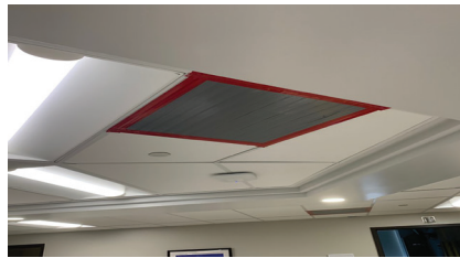
FIGURE 1 Conversion of a typical medical-surgical patient room to a temporary negative pressure patient room. (Left) A typical medical-surgical patient room may be quickly converted to a negative pressure room by placing portable HEPA exhaust fan units that are exhausted through windows directly by or via flexible duct through a fixed window panel. (Center) In this case, the return air grille is sealed. (Right) A digital pressure gage with audible alarm is placed outside the door.
